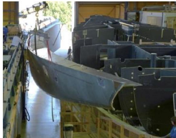
Figure 6: Hull construction of the Pink Gin VI [5]
