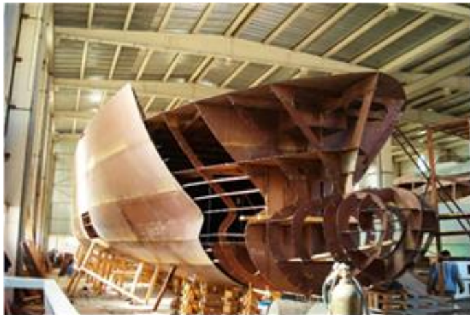
Figure 2: Illustration of the panel-block-assembly method
