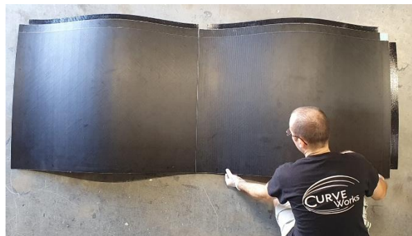
d: Alignment of two curved panels along the short sides
